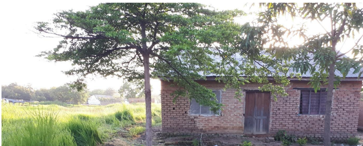
A typical example of improved housing beside a mosquito-producing rice field in rural Tanzania, constructed using bricks, timber and iron sheeting plus netting screens fitted over the windows.
